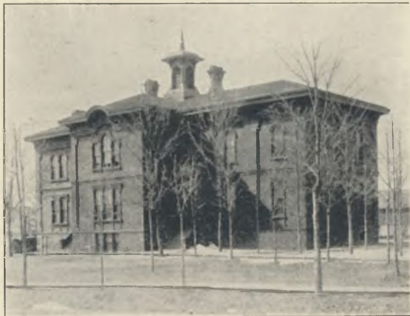
SCHOOL BUILDING DESTROYED BY FIRE
